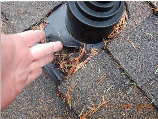
1.2 Item 2(Picture) Flashing damage
