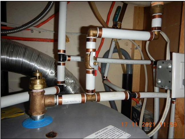
11.0 Item 4(Picture) Copper/PEX plumbing
