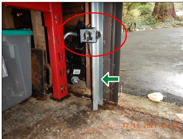
5.6 Item 1(Picture) Garage door sensors
