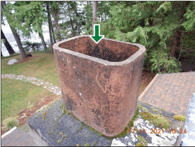
1.2 Item 4(Picture) Open flue (redundant)
