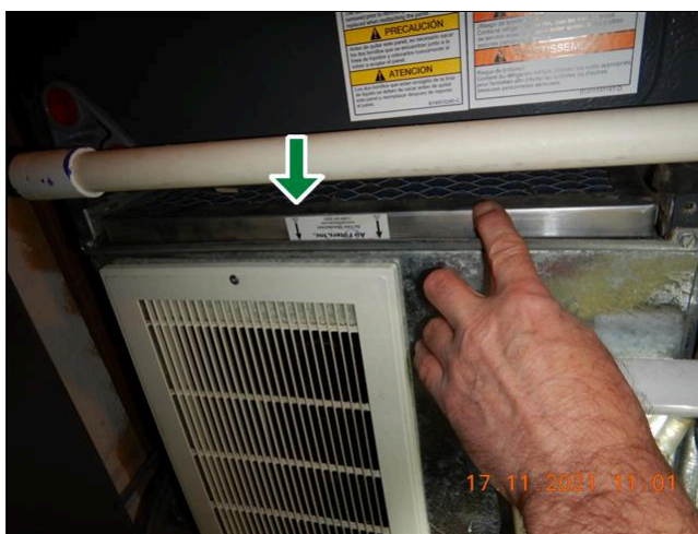
6.3 Item 2(Picture) Furnace filter
